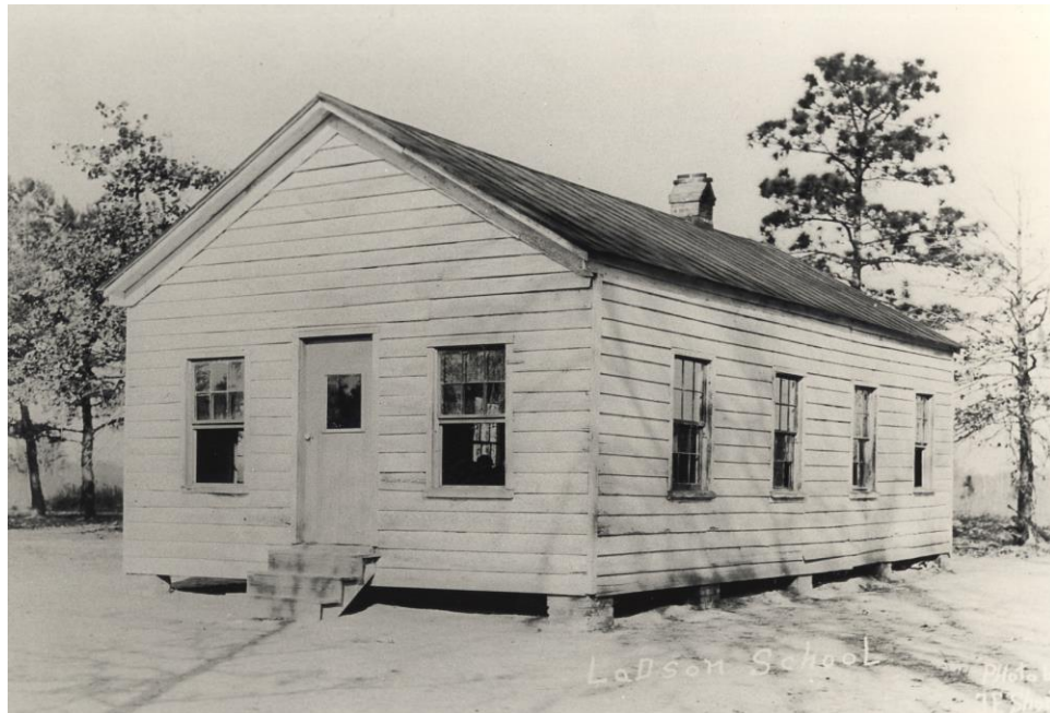
Figure 1. Ladson Elementary School, Charleston County, photograph c.1920. 11
