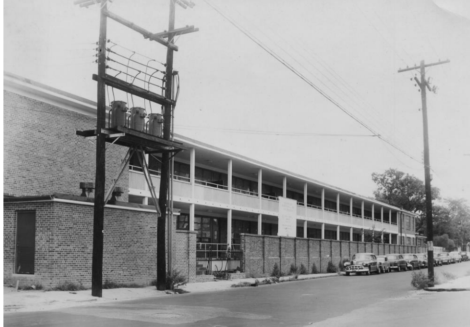
Figure 6. Memminger Elementary school, constructed 1953, showing open corridor plan. 51
