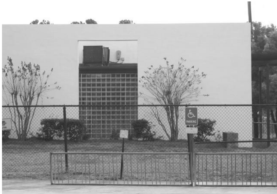
Figure 4. Murray-LaSaine Elementary, Johns Island, constructed in 1955, showing glass block windows. 46
